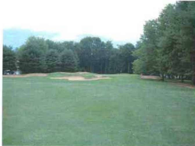
Figure 15. Rebuild the 2nd green complex
