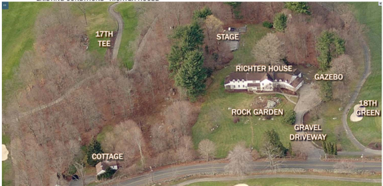
EXISTING CONDITIONS - RICHTER HOUSE
